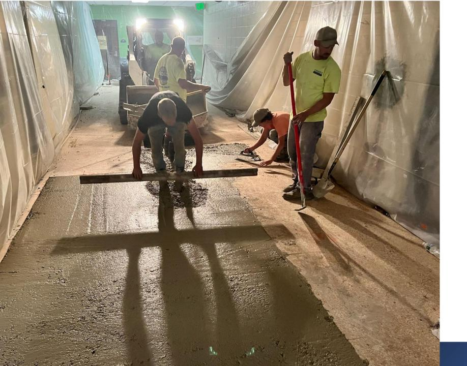
Huntertown hallway repoured after new sanitary pipes installed.
